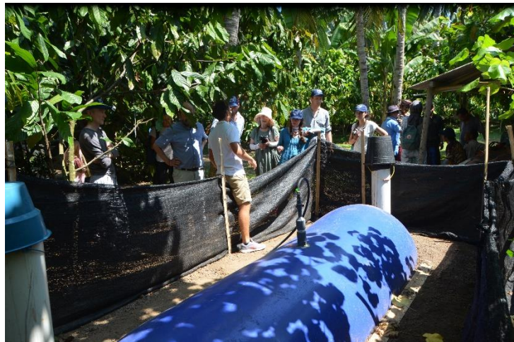
Figure 2. PVC biogas digester installation
